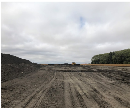
SF 49, photo facing west, one dozer pushing top soil.
