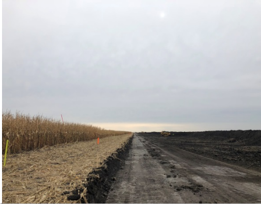
SF 49A, photo facing east, 3 dozers pushing up the remaining transition soil.
