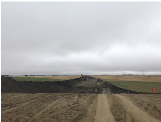
SF 44, photo facing west, 2 dozers pushing transition soil, one excavator moving soil between piles.
