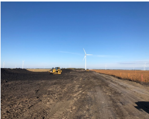
SF 48, photo facing west, topsoil stripping.
