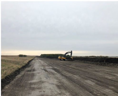
SF 49, photo facing east, one excavator separating topsoil and transition. A spotter is being used.
