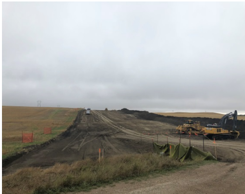
SF 44, photo facing east, one dozer pushing transition soil.
