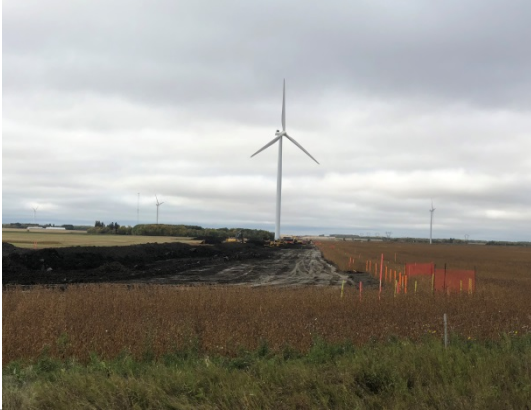
SF 48, photo facing west, multiple dozers and excavators pushing top soil to the side of the ROW.
