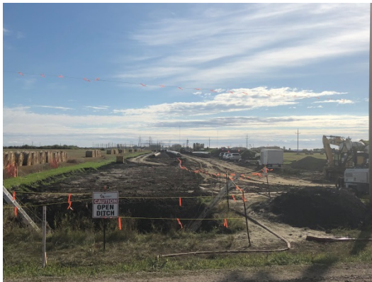
SF 19, photo facing west, crews working on pipe.
