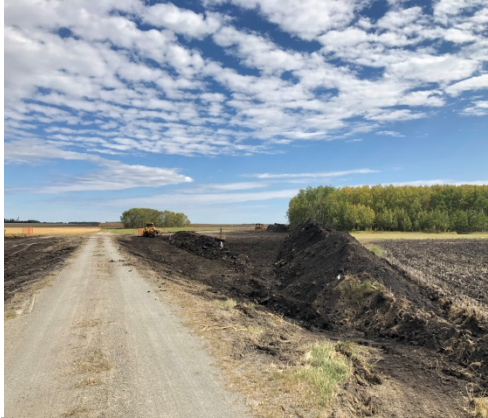
SF 49A, photo facing north east, dozers pushing topsoil, there is a grader and 4 more dozers around the corner.
