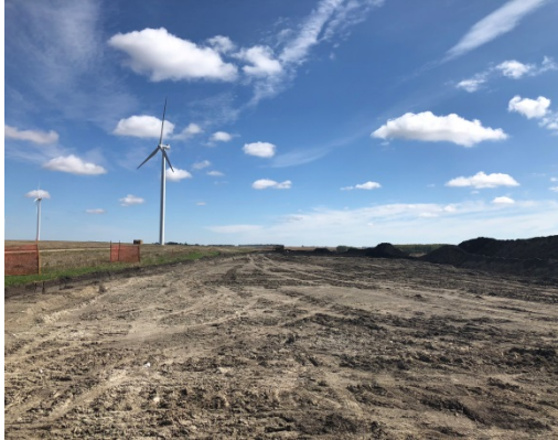
SF 49, photo facing east, 3 dozers pushing top soil, one excavator moving top soil, one grader grading the ROW.
