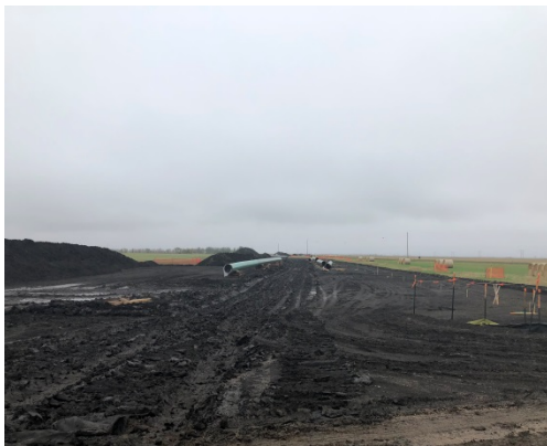
SF 24 A, photo facing west, one crew was spray-painting markings onto the pipe, there on the right hand side it's hard to see, you can also see how muddy the ROW is.
